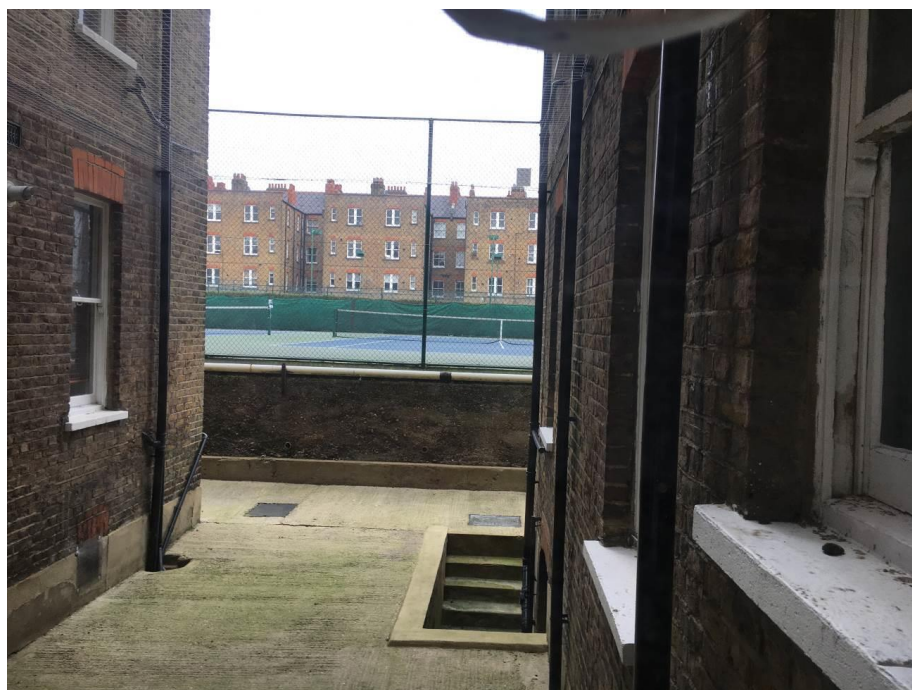
View from ground floor rear elevation window at Delaware Mansions
