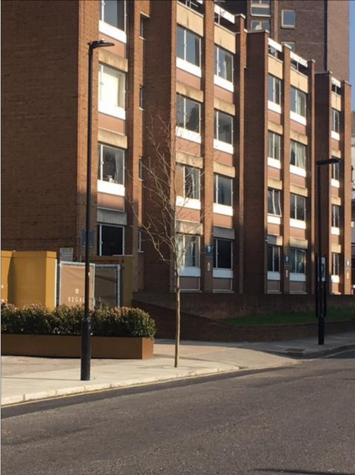
Existing Lodge Road elevation
