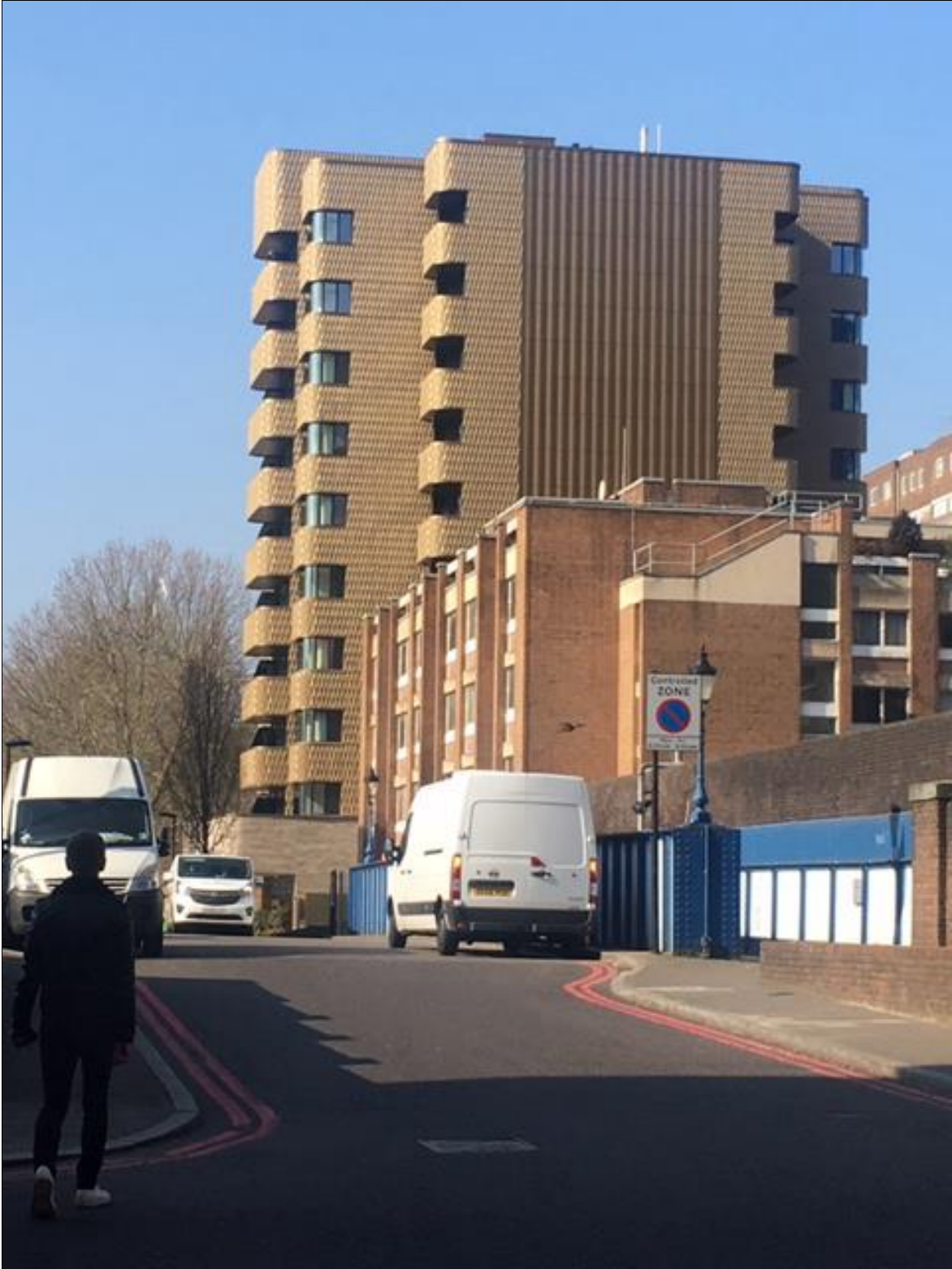
Existing Lodge Road elevation
